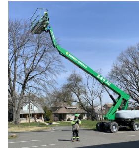
Boom Lift delivered for Steeple repair
